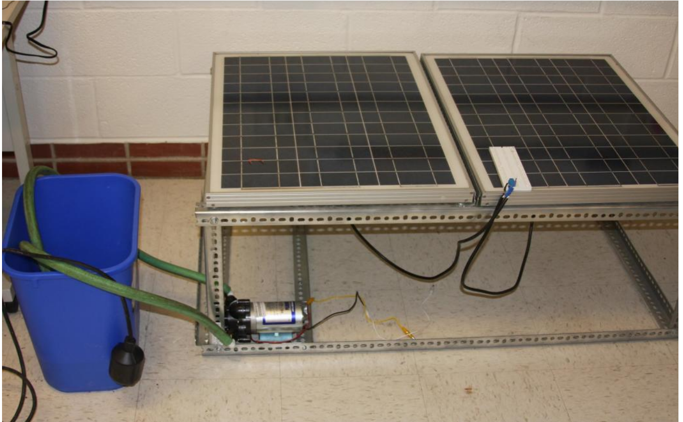
Fig. 13: Receive side solar panels and pump
