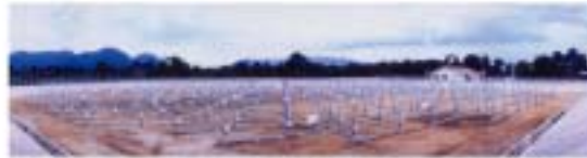
Antenna field (110m in diameter)
