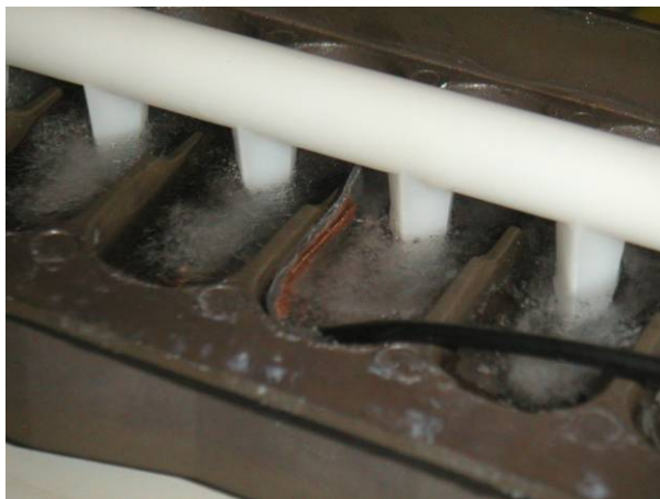
Photo 4. Water in cavity is frozen.
