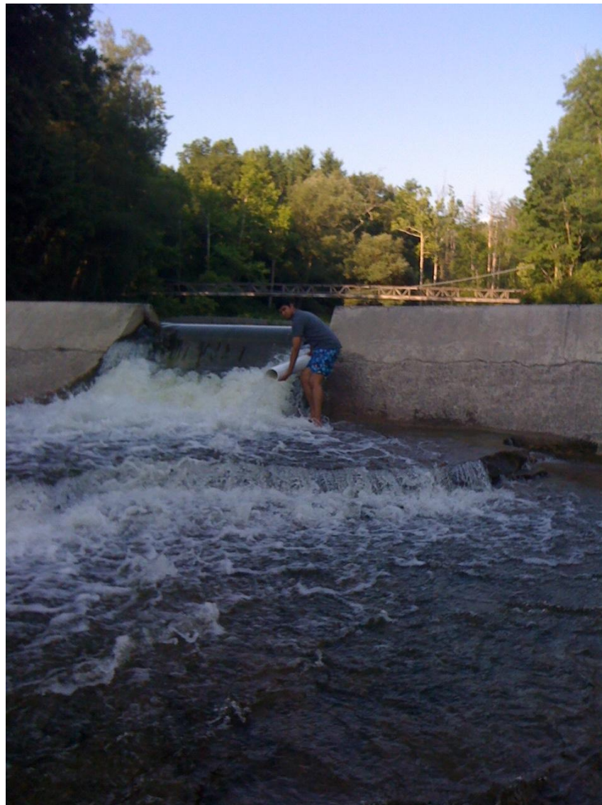
Figure 13 Water flowing through Pipe at Gorge
